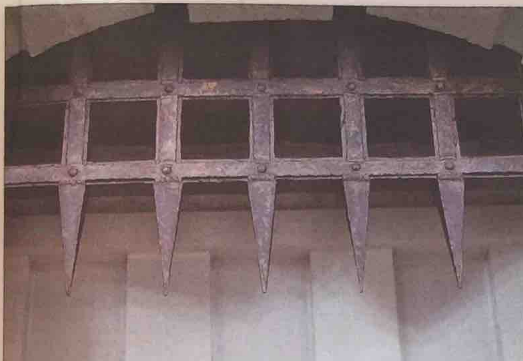
The portcullis, which hangs above the castle's front entry, is made of reclaimed oak covered with hammered metal. Portcullises in medieval castles were designed as a last line of defense.
